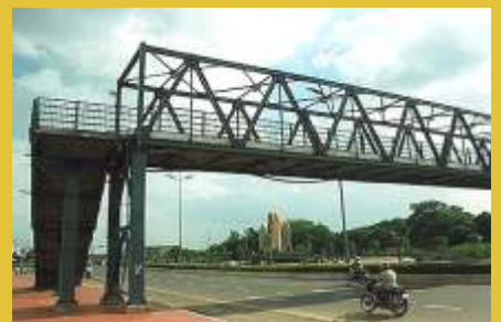
Foot Over Bridge
