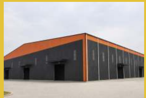
MG Contractor (BHEL Fabrication Unit)
