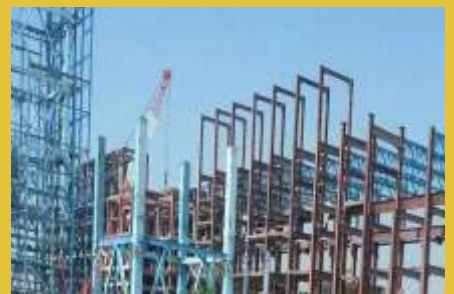
Power Plant Structure
